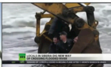
Excavator river crossing
